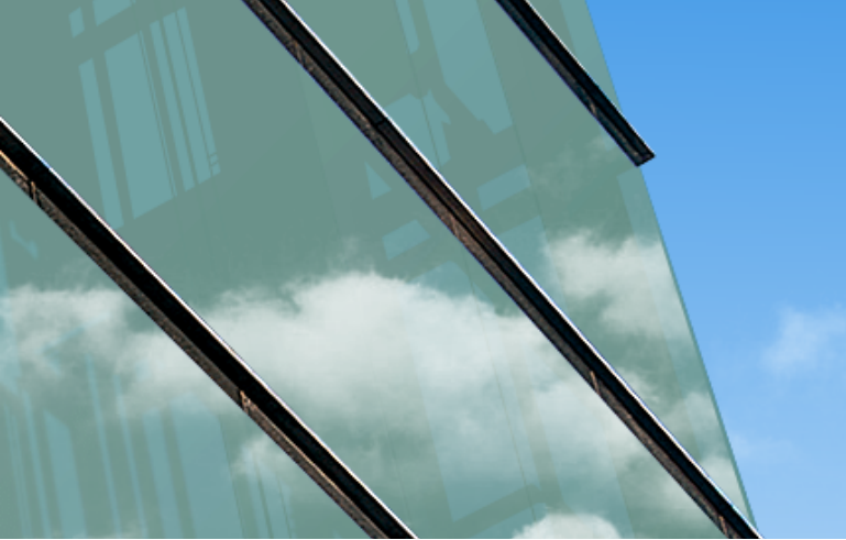
EG01 GLAZING GREEN TINT TRANSLUCENT GLAZING U-VALUE: 3.7 SHGC: 0.39
