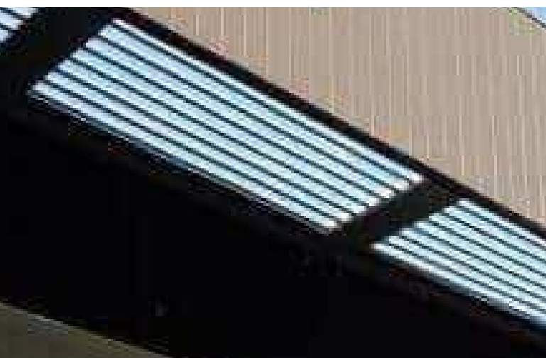
EG01 GLAZING GREEN TINT TRANSLUCENT GLAZING U-VALUE: 3.7 SHGC: 0.39
